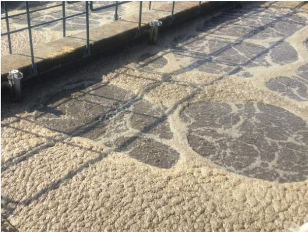
*Example light form of fine bubble aeration, with foaming*
