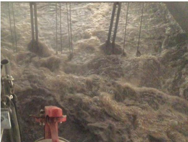
*Example coarse bubble aeration, partly to keep membranes clean*
