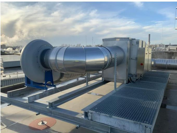
*Example WWTP Boxtel: test set-up air failure with air filters and Uvc treatment.*
